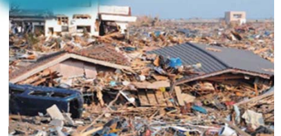
Status of housing damage (Ukedo district, Namie Town)
