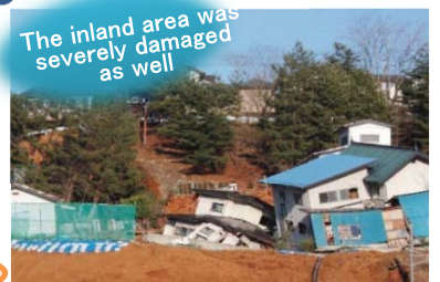
Status of housing damage (Fushigami, Fukushima City)
