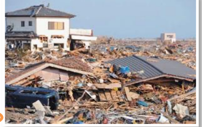
Extensive damage caused by Tsunami
