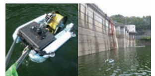
Investigation for dam wall construction with underwater robot
