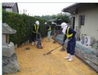
Decontamination work for housing
