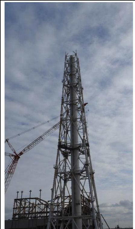
The exhaust stack has five blocks removed. A red crane is visible on the left side, and the sky is overcast with grey clouds. |
