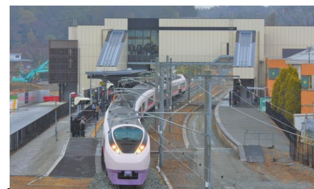
JR Joban Line resumed full service on 14 Mar. 2020
