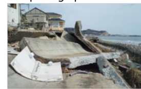
Iwaki City: Levee
