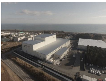
Temporary incineration facility at Okuma
