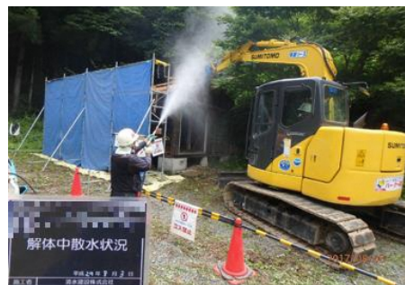
Dismantling of a damaged house
