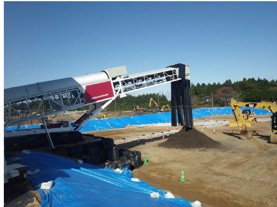
Soil Storage Facility (in Okuma)
