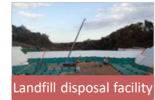
Landfill disposal facility
