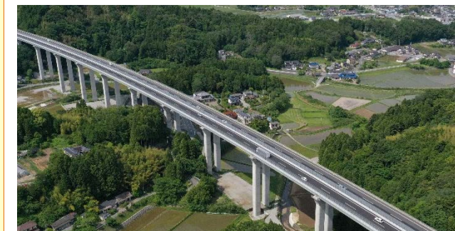
Joban Expressway (Iwaki Chuo IC- Hirono IC) A four-lane operation started on 13 Jun. 2021
