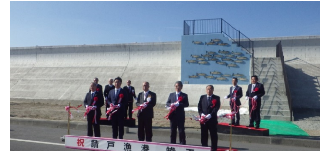
Ukedo Fishing Port completion ceremony was held on 20 Nov. 2021 Restoration of 10 fishing ports in affected areas has been completed
