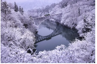
Tadami Line railway facilities
