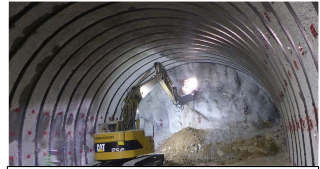
The Sekiba Tunnel in the Kawamata Town section on the National Road Route 114 was opened on 2 Mar. 2022
