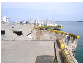
Disaster situation at Soma port(top) before and after restoration(right)
