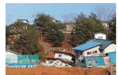
Status of housing damage (Fushigami, Fukushima City)
